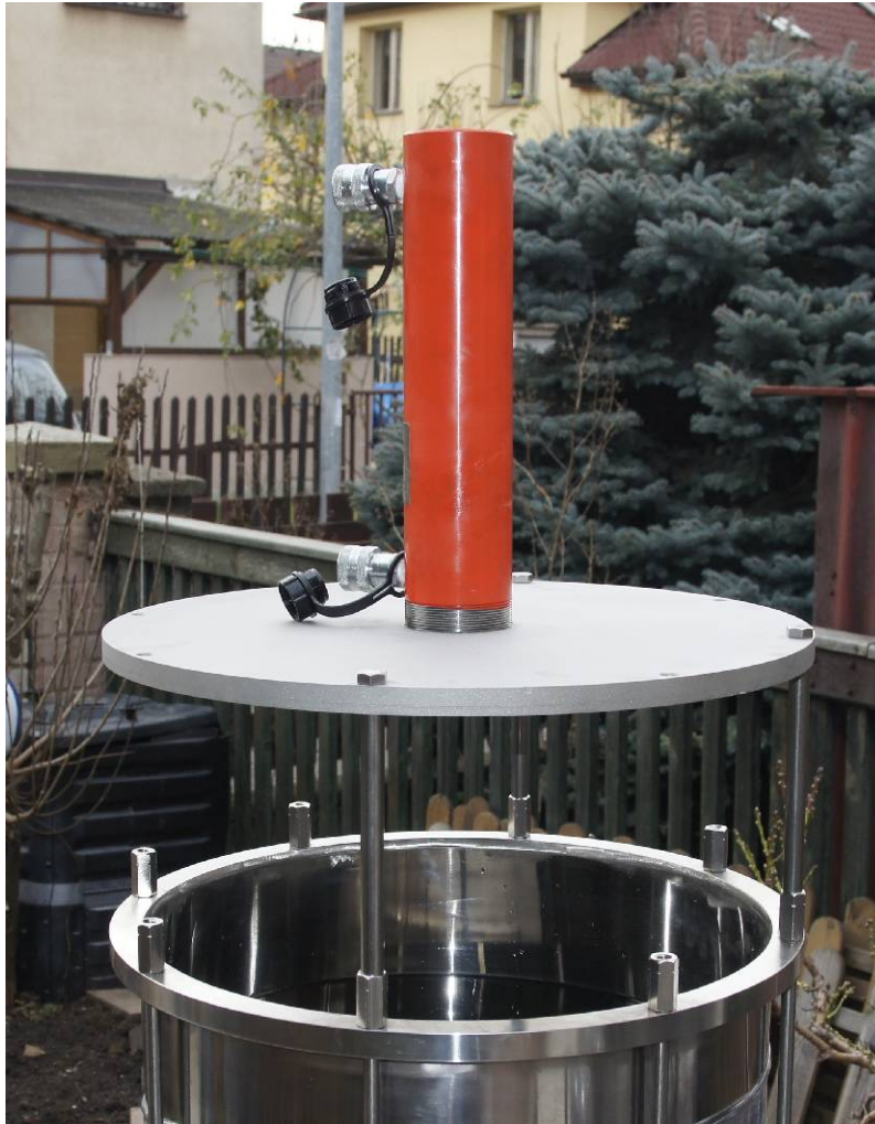
Fig. 12: Upper flange installing
